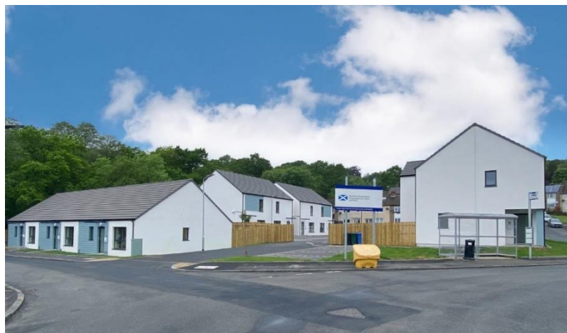
The completed new build at Linn Way, Garelochhead
